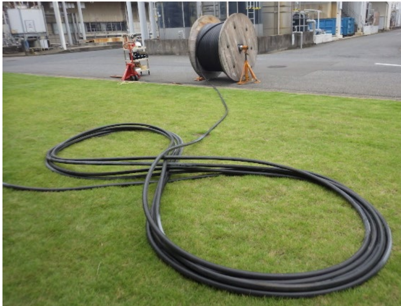
I/O WTC Deployment
