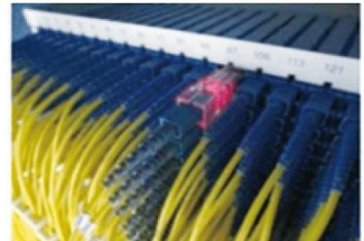
Prevention of Incorrect Removal through Transparent Connector Adapter
